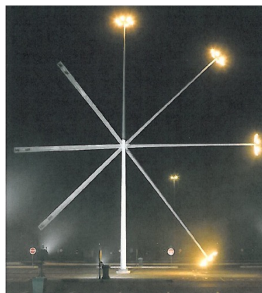
Figure 15: Scissor Mast
